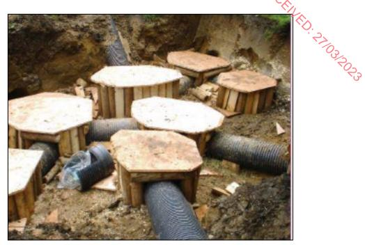
Figure 5-15 An example of an artificial sett under construction with pipe tunnels and 7 chambers (Extracted from NRA (now TII), 2005b)
